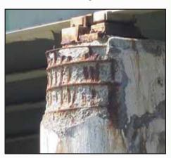
Fig 1. Cracking and spalling of concrete due to rebar corrosion
